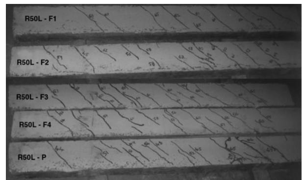
Figure 4. Tested longitudinally over reinforced beams
