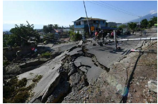
Figure 10. Damage to Roads due to Fault Rupture and Liquefaction, Palu Earthquake [15]
