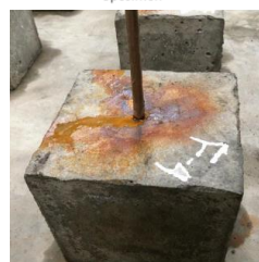
Figure 6. Potential Reading and Typical Visual Appearance After Initial Corrosion
