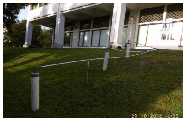
Figure 1. The Condition of the Monitored Slope at UMY Campus
