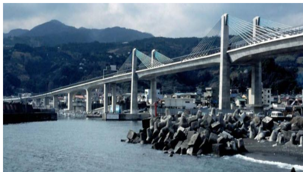
Figure 10. Odawa Blueway Bridge in Japan (Courtesy of Sumitomo Mitsui, Japan).
