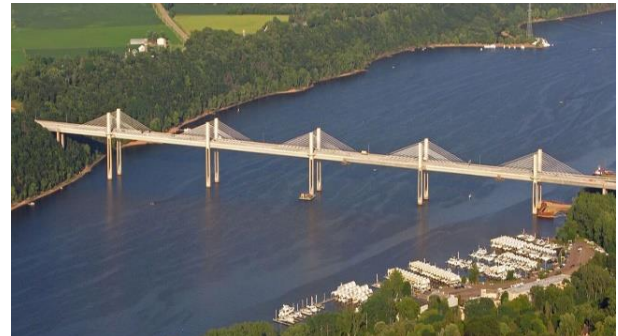
Figure 12. St. Croix Crossing Extradosed Bridge (Courtesy of Minnesota Department of Transportation)
