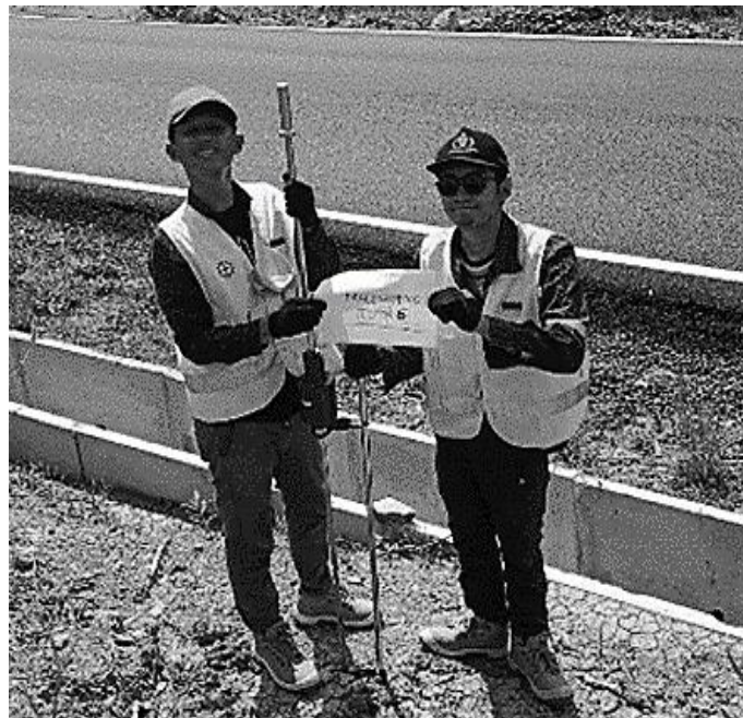
Figure 3. Dynamic Cone Penetration (DCP) Test at the Observed Location
