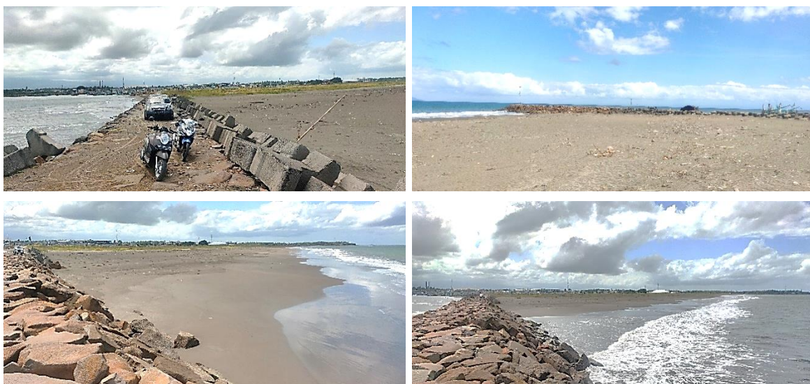
Figure 26. Coastline Survey on The Beach of Pengambangan Fish Harbour, Jembrana Regency
