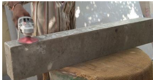
(a) Grinding of Concrete Surface
