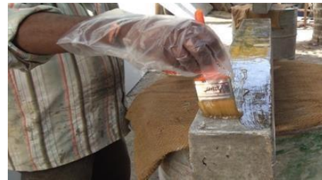
(b) Application of Epoxy Resin
