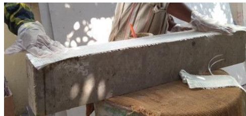
(c) Laying GFRP Layer
