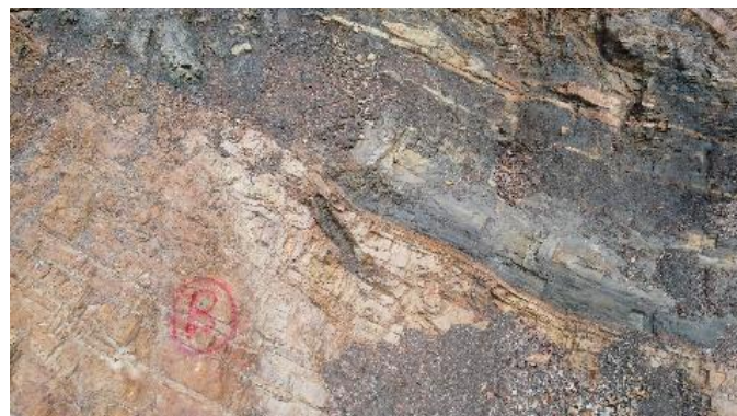
Figure 4. Ground Control Point (GCP) marked on the Slope Surface
