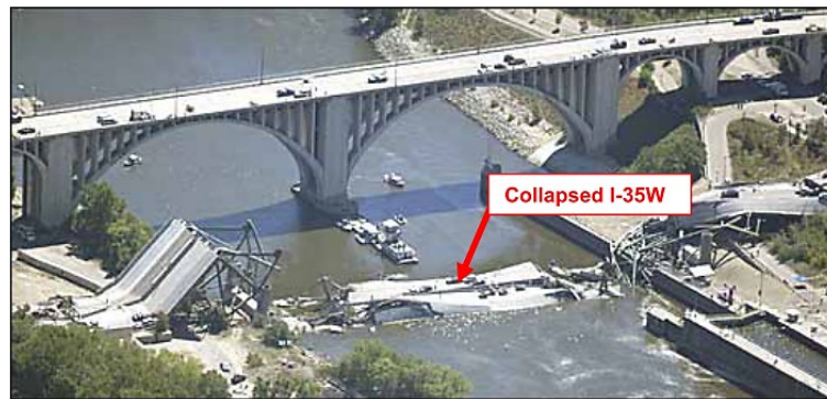
Figure 2. Photograph of the I-35W Bridge Collapse [2]
