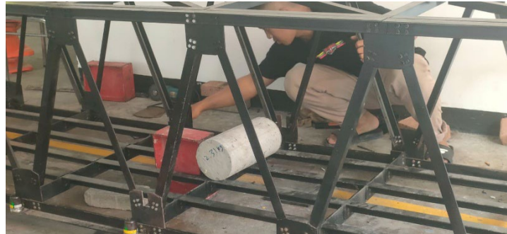
Figure 12. Experimental 10% Tearing Damage on Gusset Plate at Mid-Span
