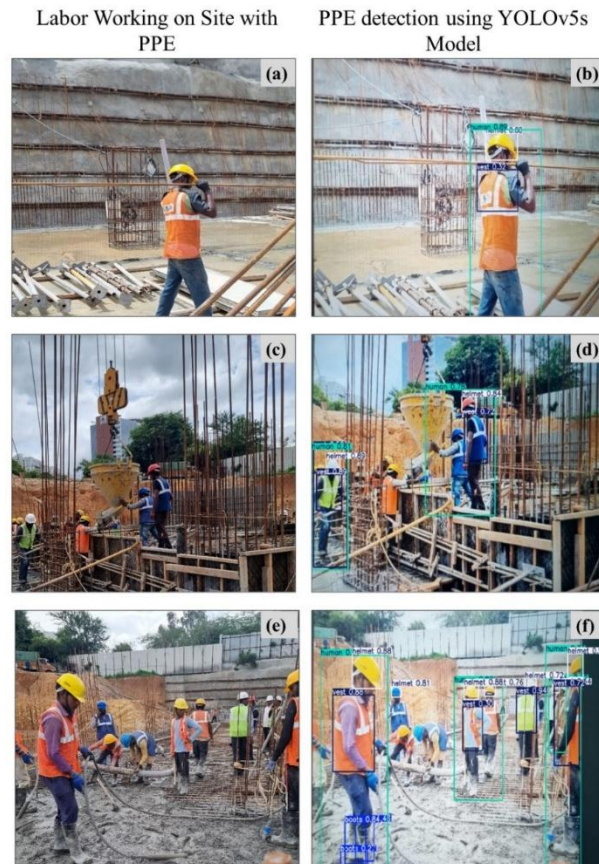
Figure 2. (a) Single Worker Carrying Rebar, (b) YOLOv5s Detection Output Showing Identified Helmets and Vests with Confidence Scores, (c) Multiple Workers at a Reinforced Concrete Pouring Site, (d) YOLOv5s Detection Output Identifying Helmets and Vests with Confidence Scores, (e) Multiple Workers Engaged in Concrete Placement, (f) YOLOv5s Detection Output Highlighting Helmets, Vests, and Boots of Multiple Workers with Confidence Scores
